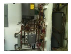
Zilmet flat expansion tanks also include a union with a double service check. This streamlines the installation process by eliminating the need for extra components and it makes it even easier to squeeze the tank into a tight spot.
