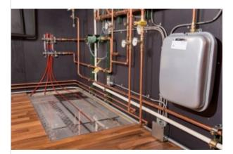
Able will be stocking 2.1- and 4.8-gallon models. The former has a depth on 3.7" while the latter clocks in in at 6.2". Have you ever seen a 5-gallon expansion tank that was only half a foot from front to back? Zilmet flat tanks are the perfect size to complement condensing boiler installs.
